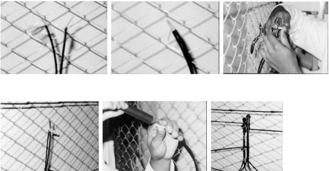
**Fig. 24, 25, 26, 27, 28, 29 – Empalme de cable microfónico**
